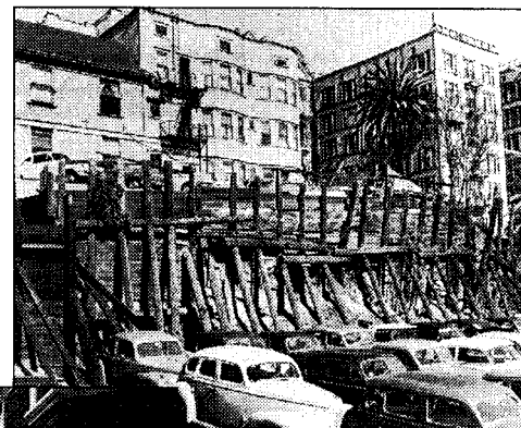
Makeshift retaining walls.
